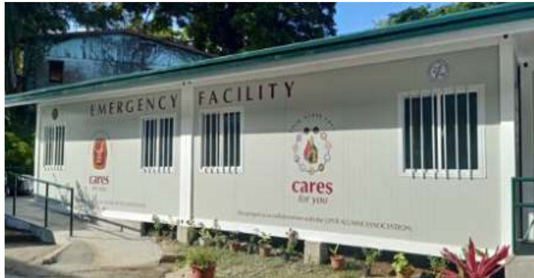
UHS Emergency Room Extension Facility
